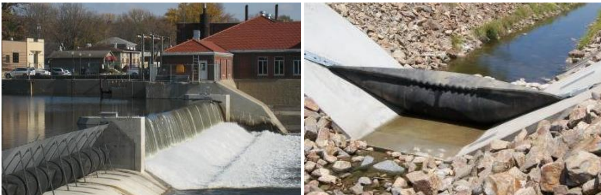
Figure 12. Inflatable rubber weir with steel gate (left) and without (right). ( Source: Obermeyer Hydro, Inc. )
