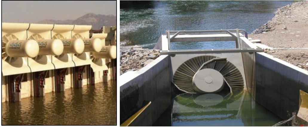
Figure 11. Hydropower turbine designs that eliminates the penstock. The HydroMatrix turbine module (left) is loaded on a guide rack that slides onto the face of a dam ( ANDRITZ HYDRO GmbH. Used by permission. ); the VLH turbine (right) spans the width of the intake works. ( Source: MJ2 Technologies North America. Used by permission. )
