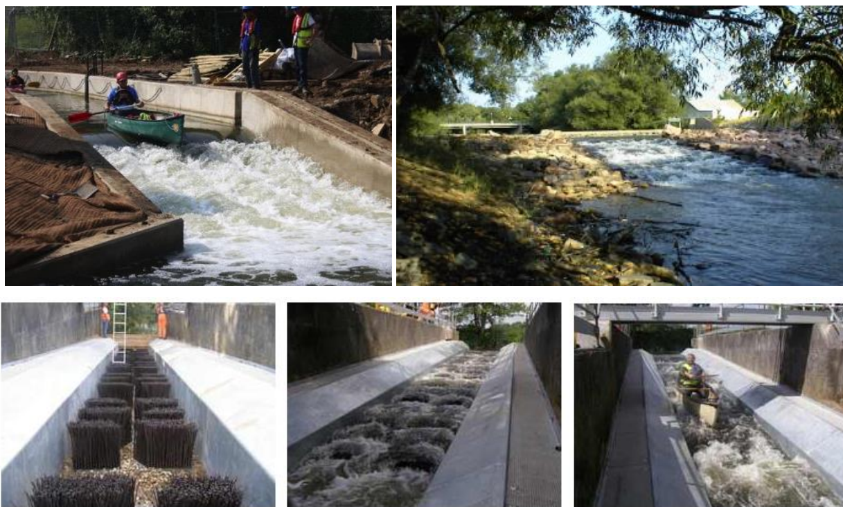
Figure 20. Combined fish passage and canoe chute on River Medway, 22 Kent, United Kingdom (top left 23 and bottom 24 ). Cache La Poudre River power plant dam/boat chute in Colorado (top right 25 ).
